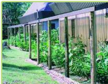
The owners of Lalati, a resort on Bega island, Fiji, wanted a wastewater system that would not pollute the water. Ecological Engineering Group designed garden-like wastewater systems that use up washwater at each building. The system also features site-built composting toilets with micro-flush toilets that are compatible with an upscale resort. Guests feel good knowing they are not polluting the island’s coral reefs which provide world-class diving.
