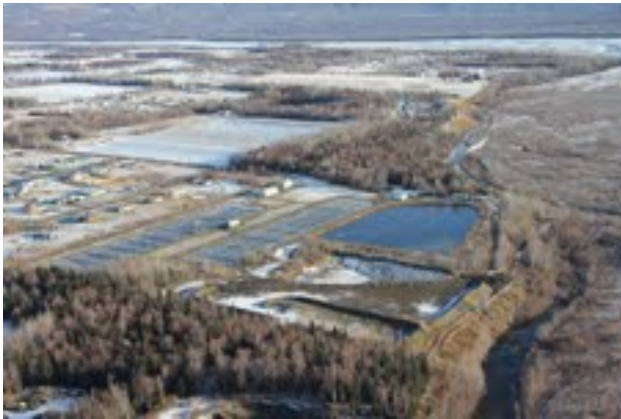
Palmer's wastewater treatment plant seen from the air.
